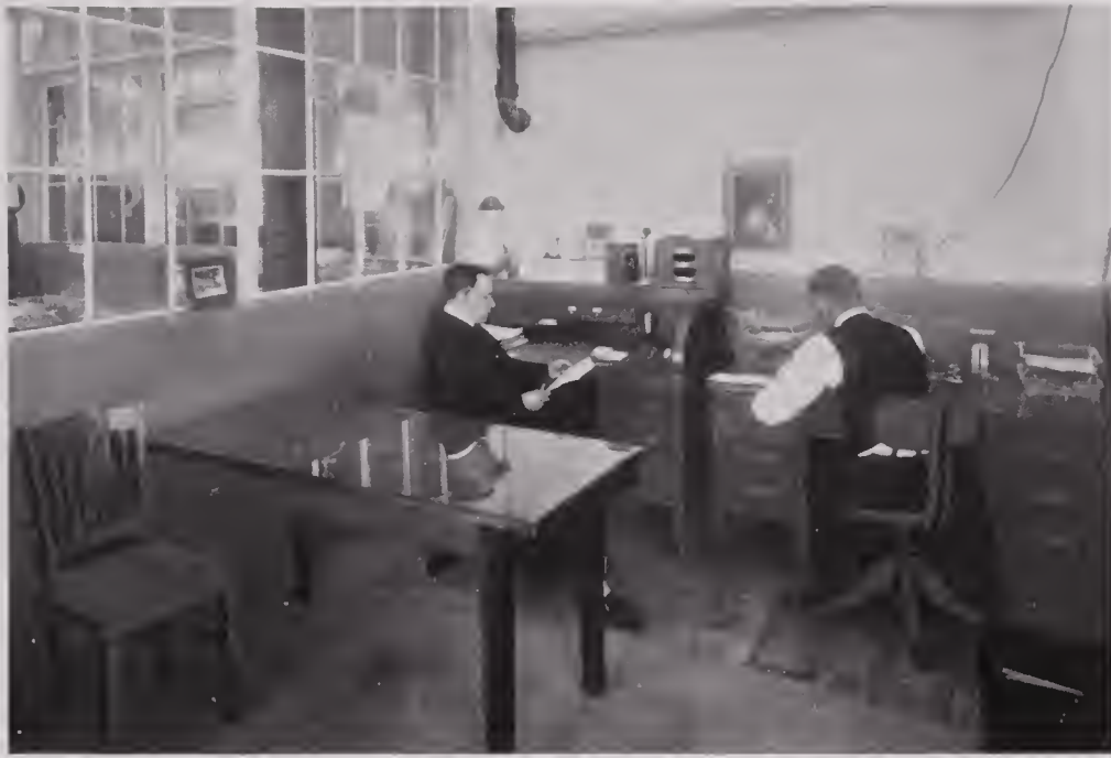
OFFICE OF WORKS MANAGING ENGINEER Factory Building Number Two
